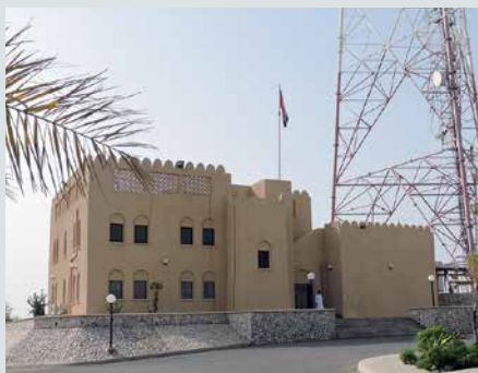
The transmitter site in Ruwi, a district of Oman's capital Muscat, is the main station of the Public Authority for Radio and Television.
